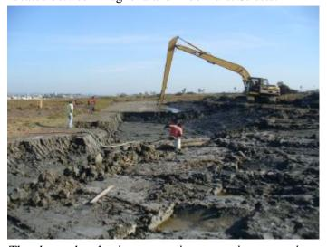
They began by clearing non-native vegetation, preparing a dewatering system and delivering equipment. The dewatering system has been installed, vegetation has been cleared and extensive excavation, grading and hauling operations are now underway.
